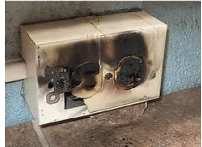
Are all outlets and switches cool to the touch? *Unusually warm outlets or switches may indicate an unsafe wiring condition exists, such as a loose electrical connection that can start a fire. (Sometimes dimmer switches may become warm during normal use).*
