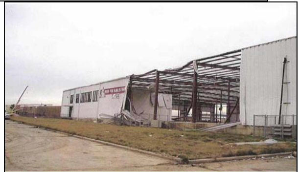
Food for families New Orleans, La Wind and water damage Hurricane Katrina
